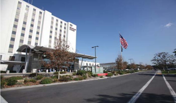
Figure 4.9: Existing view within the VA site.
